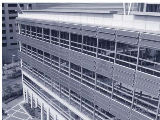
Fig. 1 Solar panels outside a building in Hong Kong Science Park
